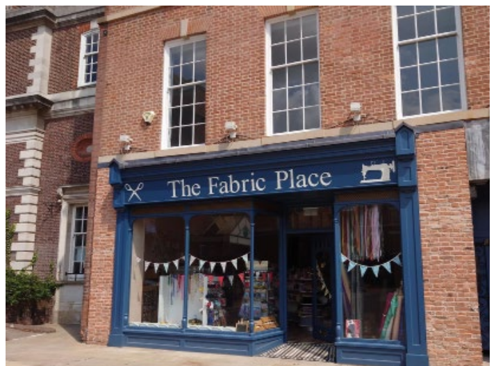
THI Gainsborough Market Place
